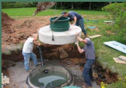
Pump station installation.
