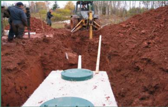
Septic tank and pump tank installation.
