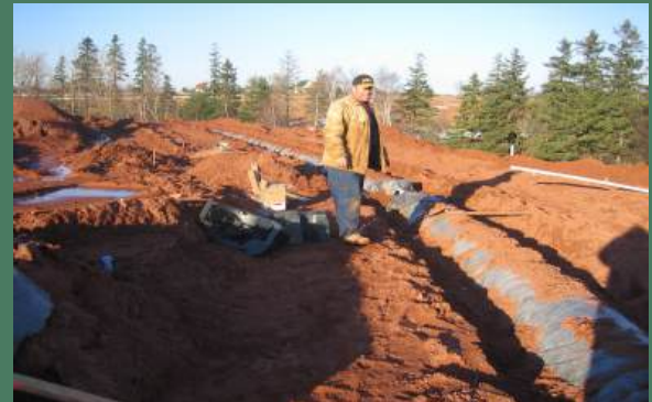
Leaching chambers installed in approved fill.
