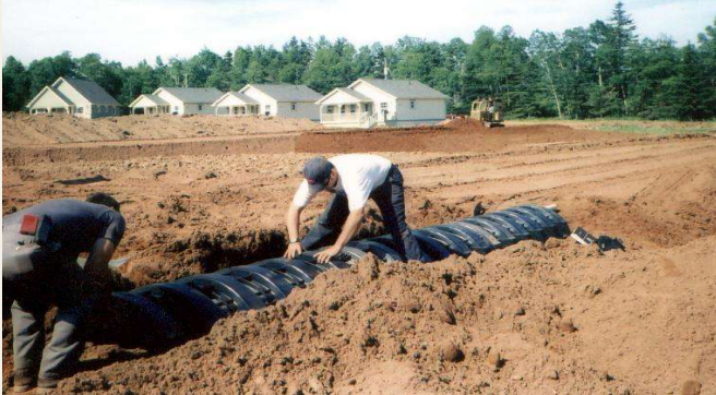
Installing Leaching Chamber Disposal Field
